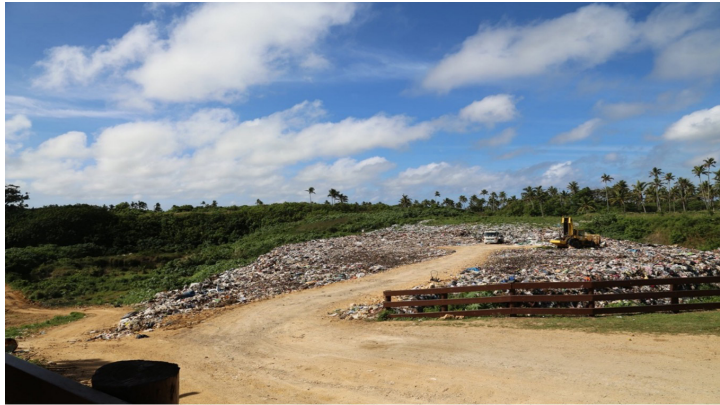
Figure 16: Tapuhia Waste Management Facility tip face, Tongatapu
