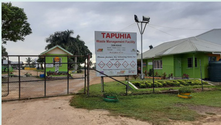
Figure 14: Entrance to the Tapuhia Waste Management Facility, Tongatapu
